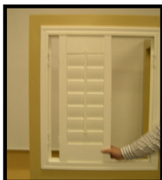
Position panel in the frame.
