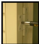
Loosen screws.
