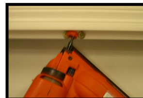
Only secure one screw into the top frame.
