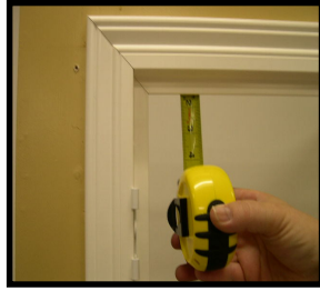
Measure Right & Top frame for spacing.
