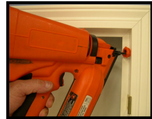
Only secure one screw into the top right frame.
