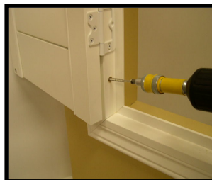
Pre-Drill bottom right & left frame.
