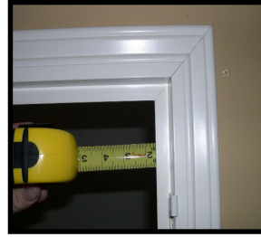
Measure Left & Top frame for spacing.
