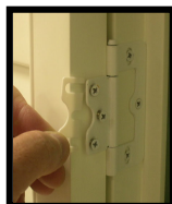
Insert spacer behind hinge.
