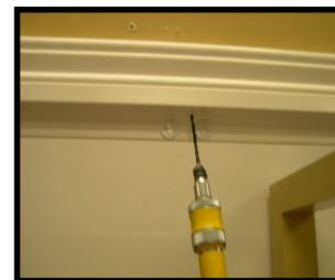
Pre-Drill middle of top and bottom frame.
