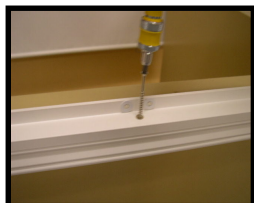
Only secure one screw into the bottom frame.
