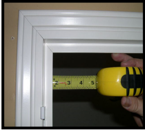
Measure Right & Top frame for spacing.
