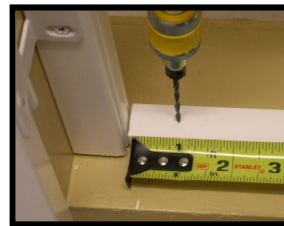
Pre-drilling is recommended to avoid splitting of the light block.
