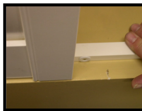
Adjust light block back or forward to bring panel flush with wall plain.
