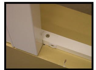
After adjustment, hold light block in place, open panel and secure the center of the light block between the magnet catch plates.
