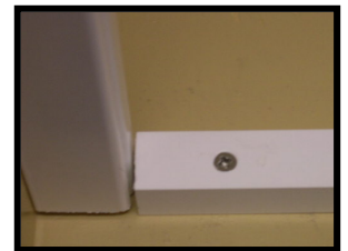
Pre-drilling is recommended to avoid splitting of the light block.
