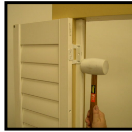
Repeat insert installation for right hang strip.
